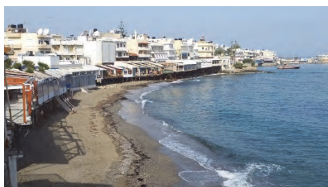
Fig.5: Coastline with tourism facilities and erosion evidence
