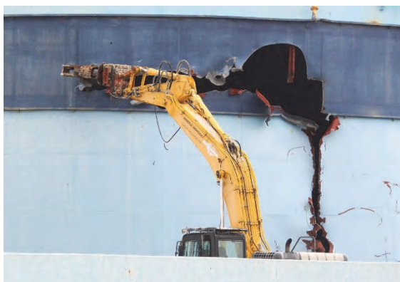
Fig.3 Demolition of storage tanks
