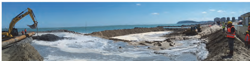
Moments of the intervention: the dredging vessel approaching the pipeline graft | a backflow yard work on the coast seen by year 2021.
